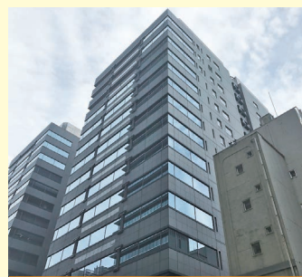
Kouwa Nishishinbashi Building - B
