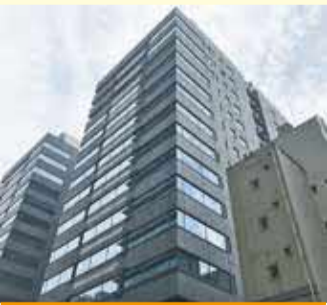
Kouwa Nishishinbashi Building - B
